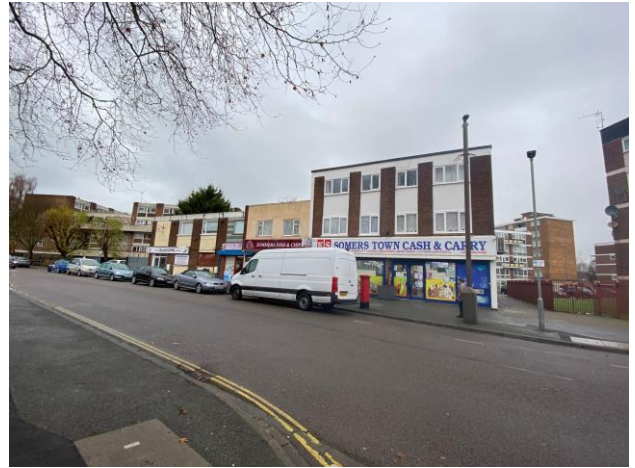
The front of the site from the north-east
