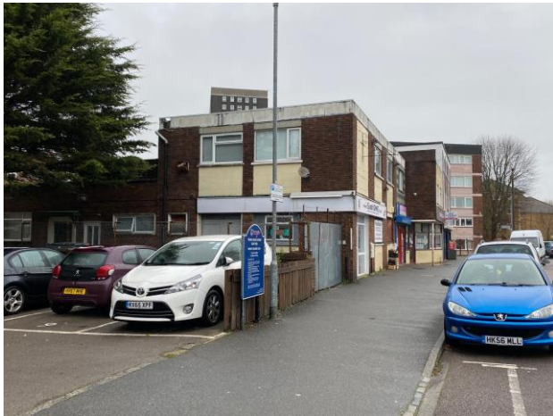
The side of the site from the south-west
